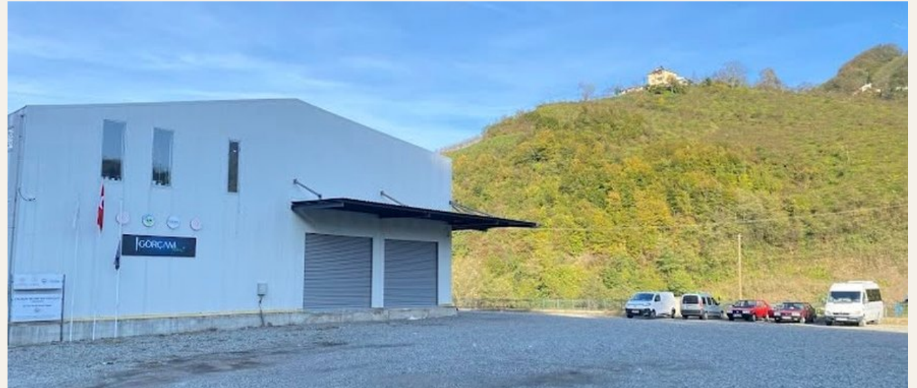
MESTIA production facility · Görele, Giresun
